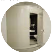
6. Main body installation completed
